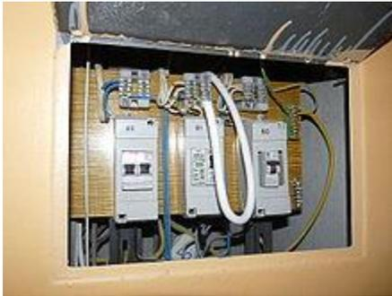
Flat 81 is waiting to be upgraded from Soviet-era aluminum cable to modern copper cable.
